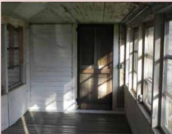
Breezeway with new siding and original floorboards. Exterior wall with new siding and repaired window frame.
